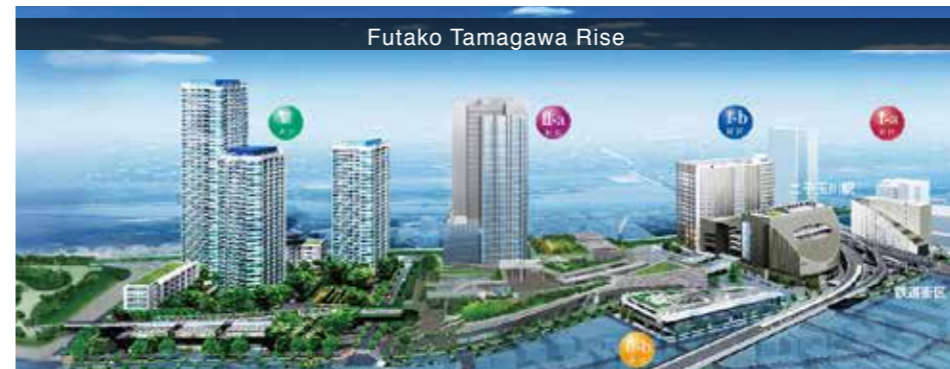
Futako Tamagawa Rise <Redevelopment Project> Management of the entire area of the condominium and commercial buildings
